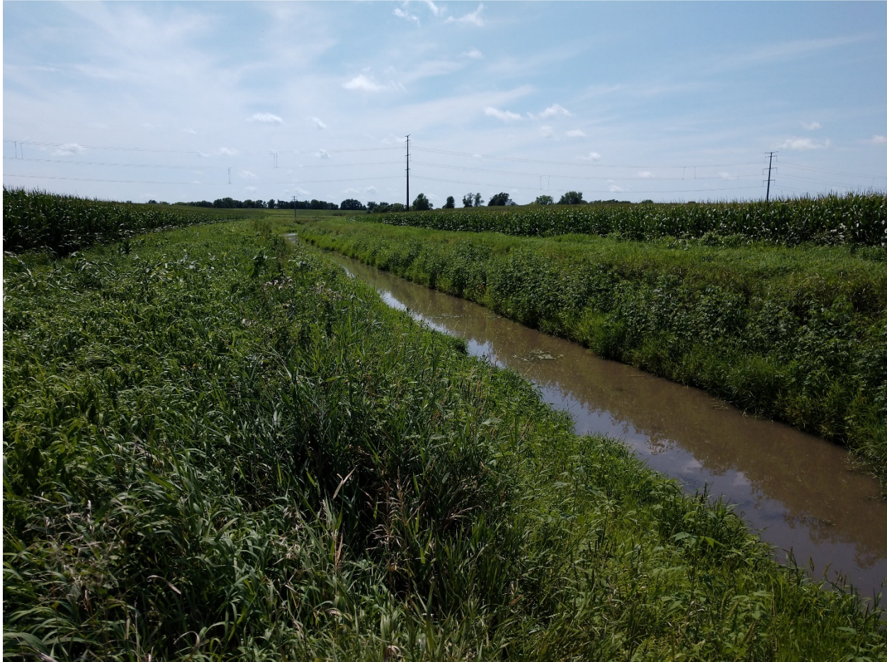
Main Line with Vegetated Buffers
